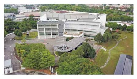
The main building, with 4,300 m<sup>2</sup> net floor area, features an innovative architectural design combining functional aesthetics with energy efficiency. The Building Energy Index (BEI) of the GEO Building is the lowest in its class, reaching an average Net BEI of 27 kWh/m<sup>2</sup>/year.
