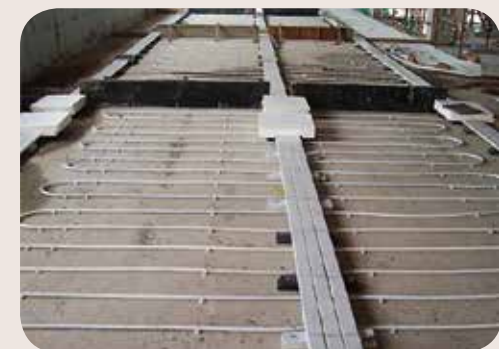
Close up view of the PEX pipes installation in Floor Slabs
