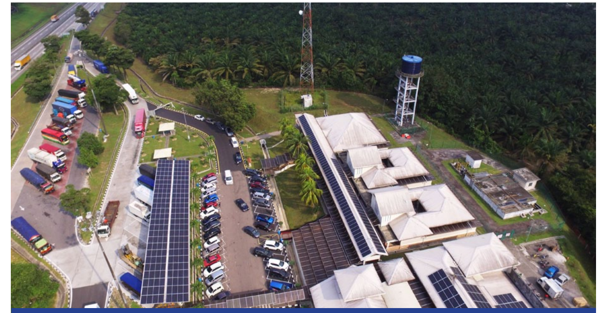
Bird's eye view of rooftop solar panels at PLUS Machap, RSA (Northbound)
