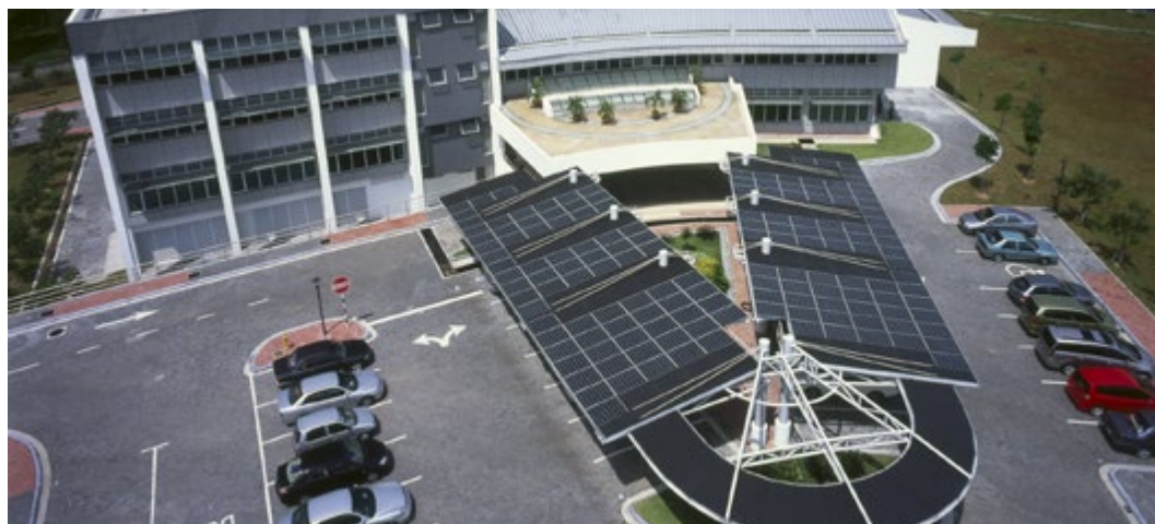
Figure 5.1: GreenTech Malaysia's Green Energy Office (GEO) Building
