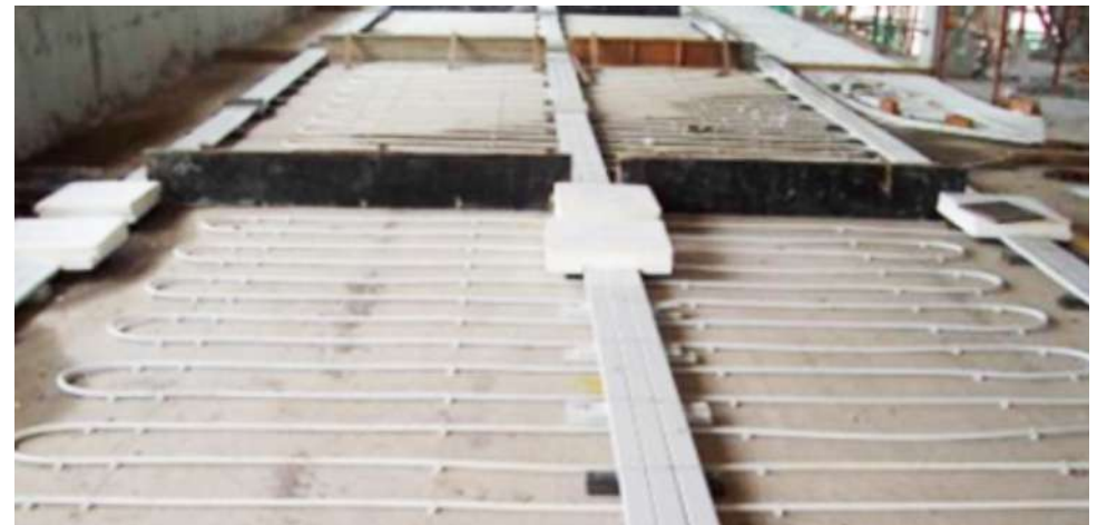
PEX Pipes Before Covered With Structural Concrete
