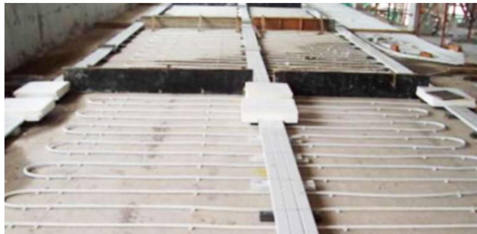
PEX Pipes Before Covered With Structural Concrete
