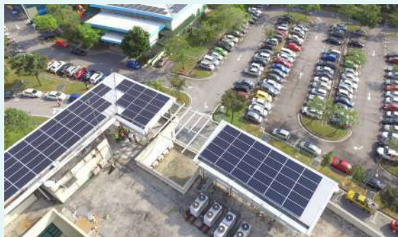
Solar PV Panels at Persada PLUS
