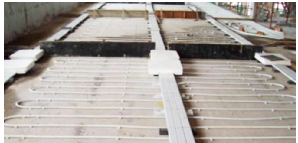
PEX Pipes Before Covered With Structural Concrete
