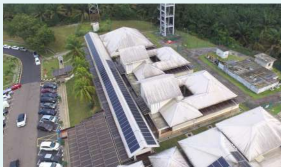
The Solar PV Panels at PLUS RSA Machap, Northbound
